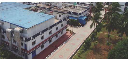
Oncology Facility SEZ Visakhapatnam, India
